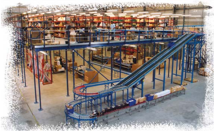
Single tier floor with conveyor access
